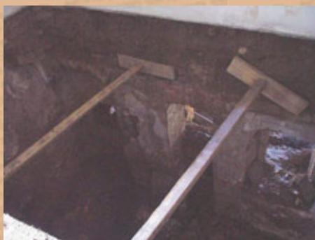
The upper picture demonstrates the view from room entrance to the right side, ceiling - floor of the room were fallen in and the opposite walls had to be braced to prevent ruining of the masonry (middle picture) .
